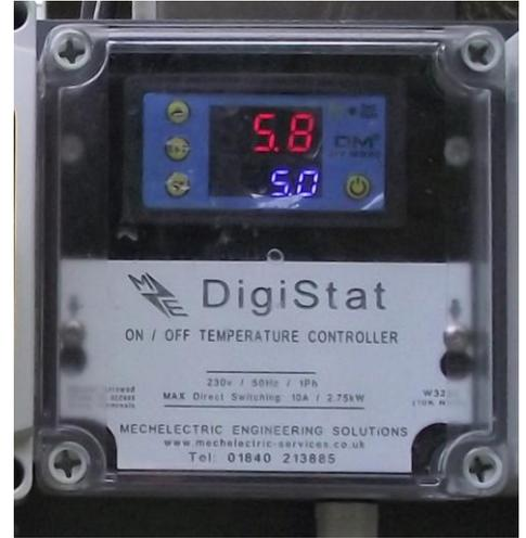
The DIGISTAT 3 is configurable for either HEATING or COOLING applications such as electrical space heaters, coolers, refrigeration, duct heaters, fan systems, air handling units, trace heating etc.
